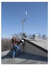
Weather monitoring specialist Glen Roebke of the HPRCC installs an anemometer and wind vane on the building in Lincoln.
